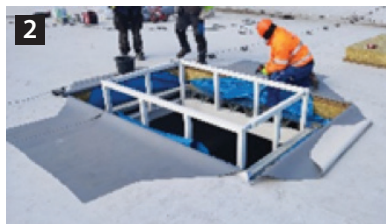
2 Installatie dak opstand in dakopening
